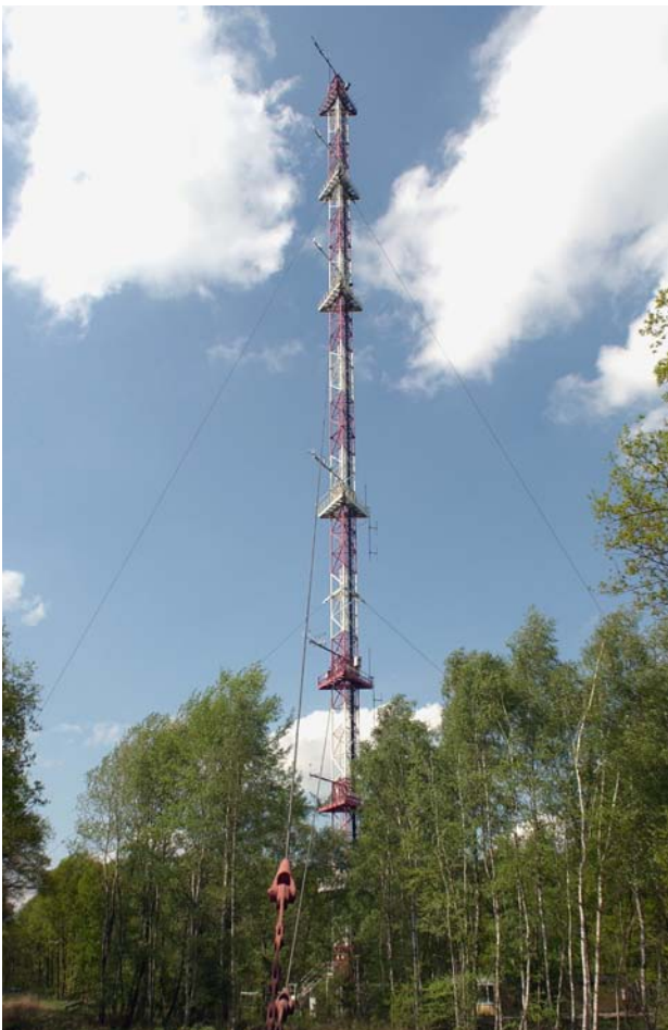
The purpose of the meteorological tower, which is 124 metres high and thus the highest structure at Forschungszentrum Jülich, is to monitor the area.
